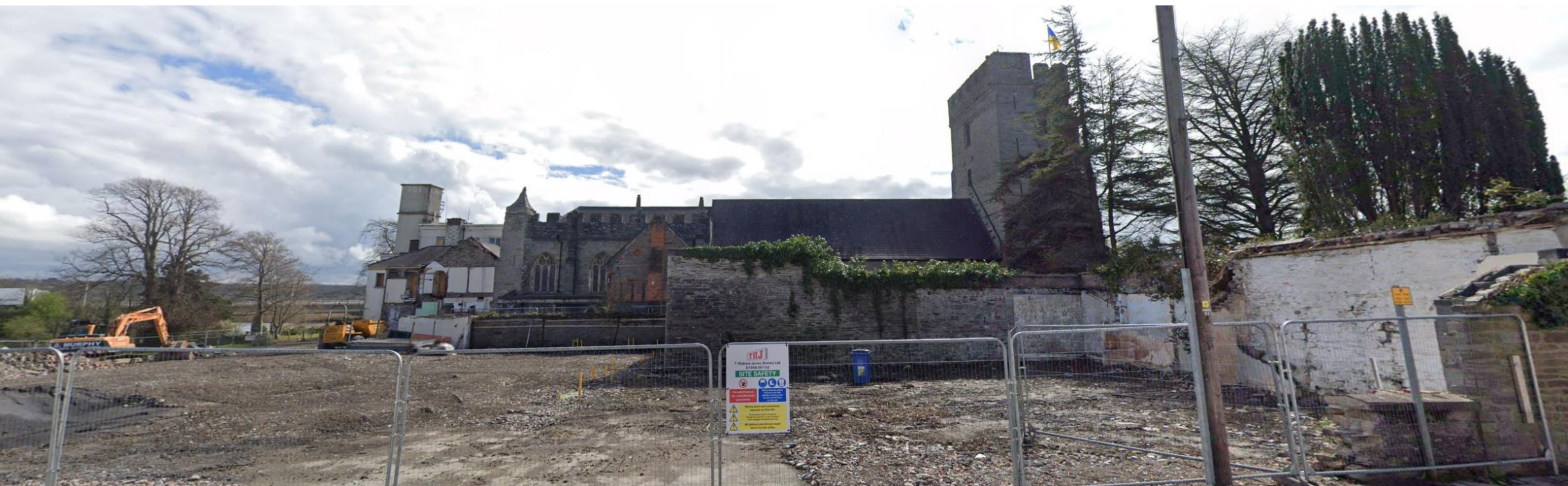
Below: Post-demolition view of the hospital and St Mary's Church as seen from Pont-Y-Cleifion.
