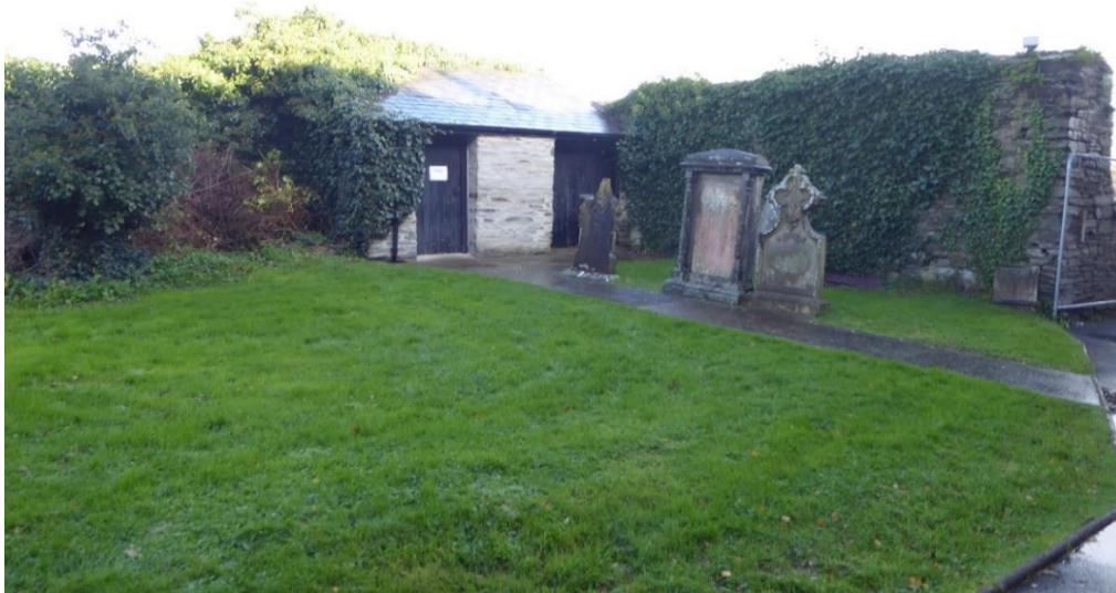
Figure 69 View from churchyard showing wall to be taken down and the monopitch building to the north
