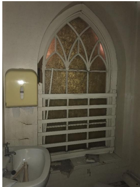
Figure 36 1 st floor upvc window in arched opening Figure 37 1 st floor sash window with intersecting glazing bars
