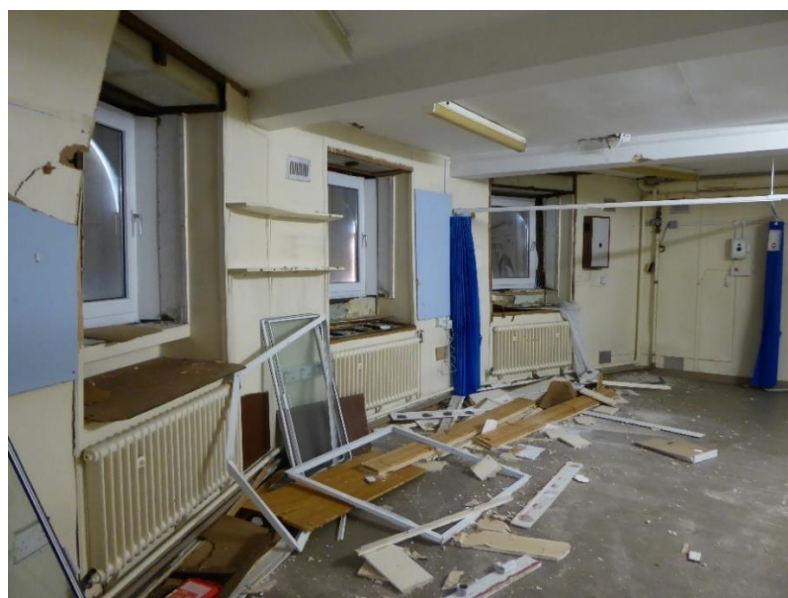
Figure 35 Basement room of original part of former Priory House
