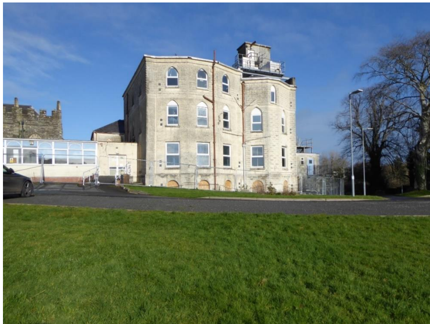
Figure 13 South front of the former Priory House as seen in 2021
