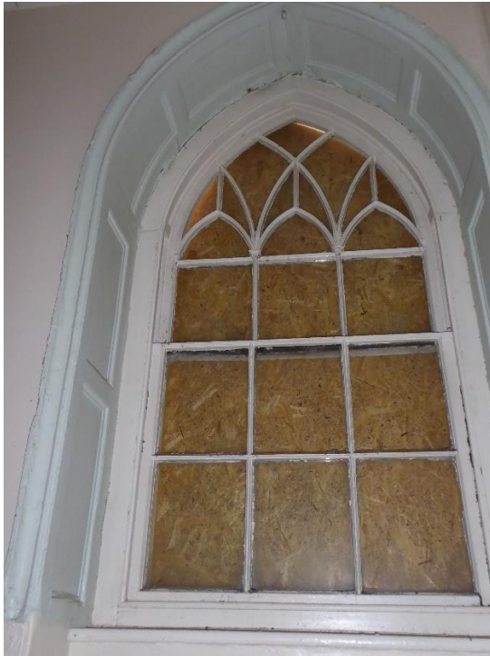
Figure 27 Window to staircase
