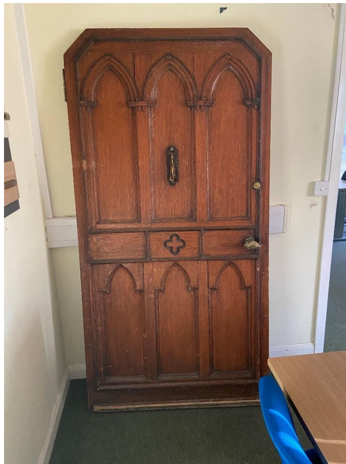
Figure 31 Former hospital main door to Priory House currently stored for reinstatement © Wales and West Housing Association
