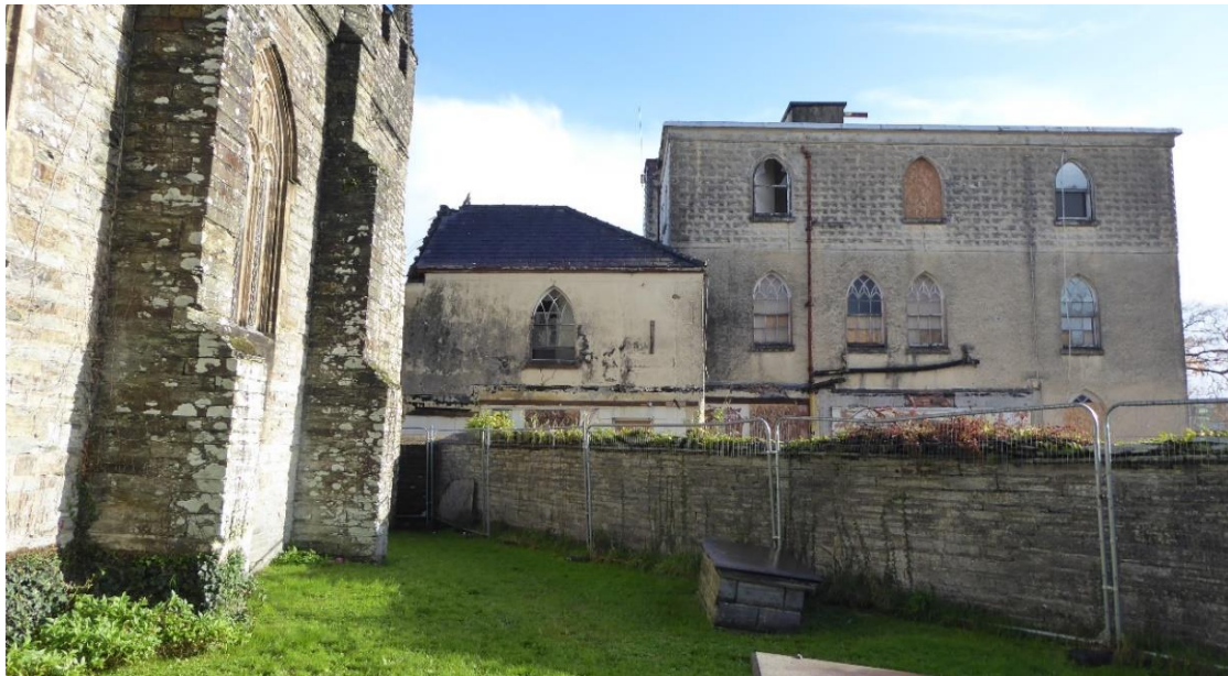
Figure 71 Existing boundary wall on diagonal line to south of chancel
