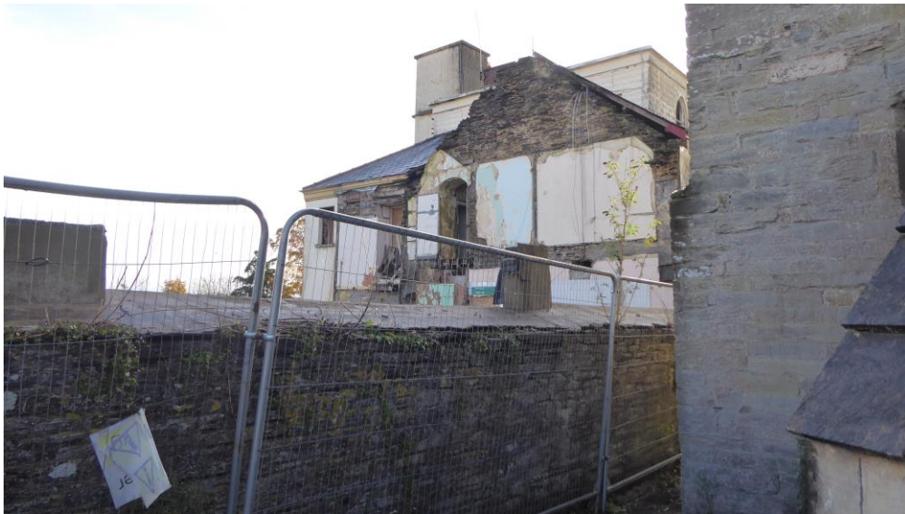
Figure 77 Existing boundary at east end of church
