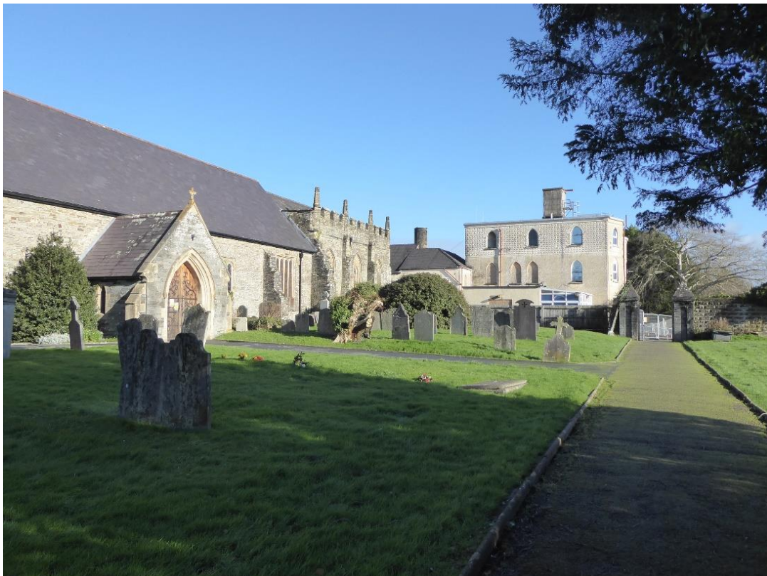
Figure 55 View towards the hospital from churchyard – a view that has been adversely affected by the hospital alterations but which will be enhanced by the proposed development
