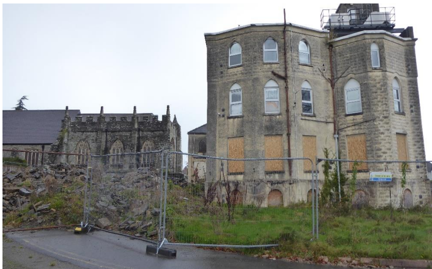
Figure 14 South front of the former Priory House as seen in 2023
