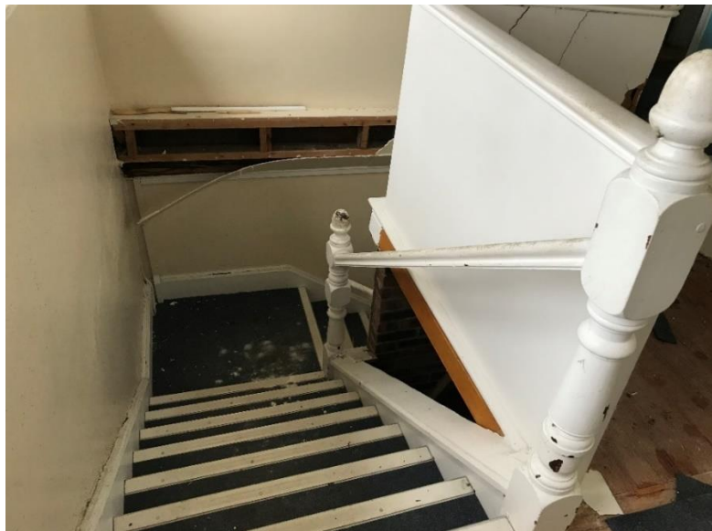
Figure 39 Stairs to 2 nd floor, view down from 2 nd floor landing
