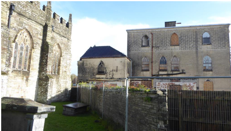
Figure 43 West elevation of Priory House seen from churchyard and south side of chancel
