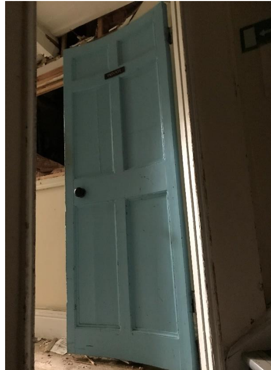
Figure 28 Curved door from staircase to service range
