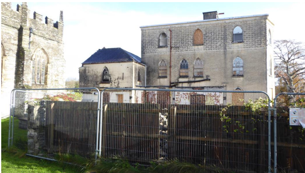
Figure 78 Existing boundary to south of the chancel
