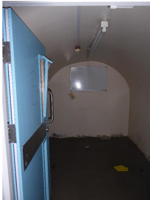
Figure 34 Basement store of former Priory House
