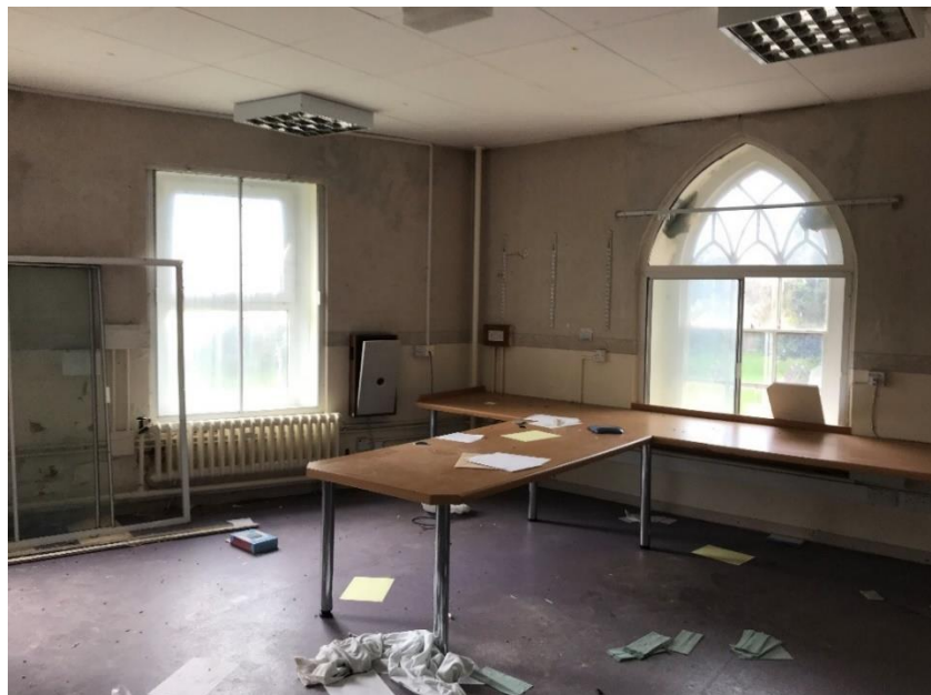
Figure 38 1 st floor room to original Priory House, SW corner
