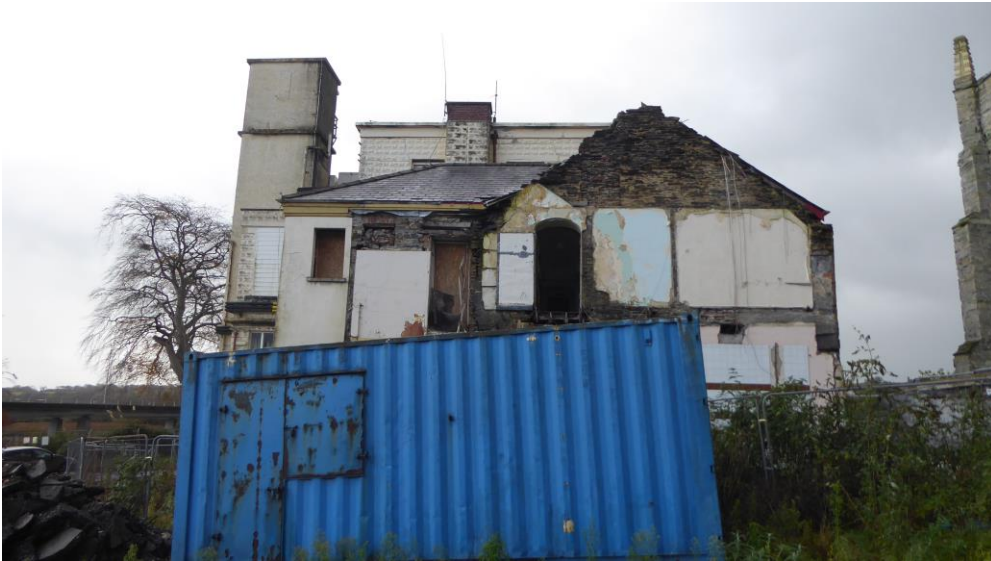
Figure 21 North side (rear) as seen November 2023 following demolition of ancillary ranges
