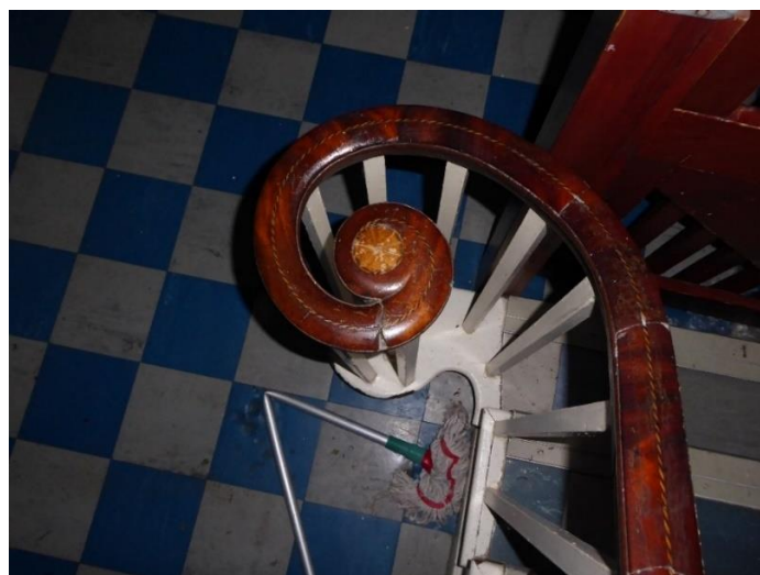
Figure 26 Inlaid handrail and scrolled newel at foot of main staircase
