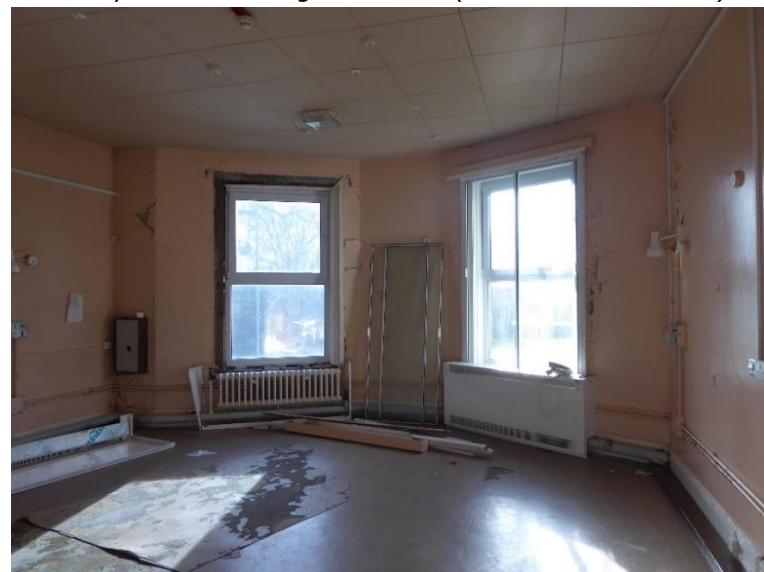
Figure 33 Former Onnen Ward in ground floor (south wall) of Priory House C20th extension
