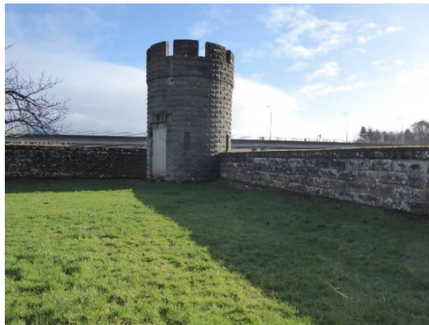
Figure 48 Round tower (part of pumping station) at south-east corner of boundary wall
