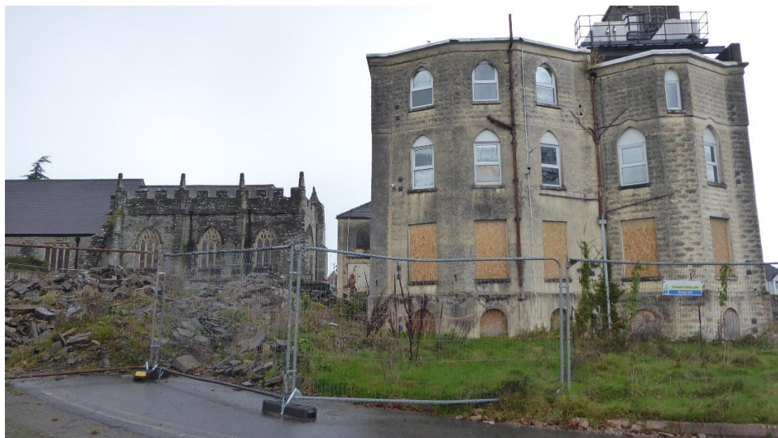
Figure 61 South front as existing showing the out of character fenestration and evidencing how the proposed changes will enhance this elevation
