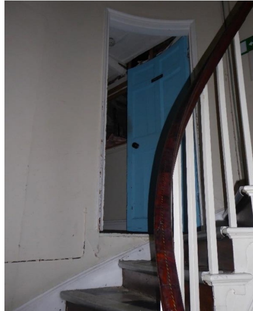
Figure 25 Staircase and door to Service Range
