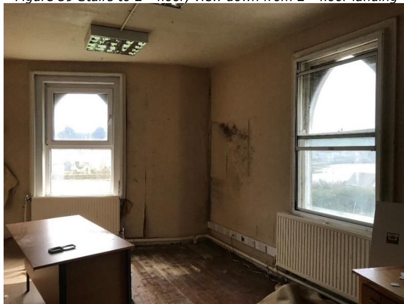
Figure 40 2 nd floor corner room to original Priory House showing pointed arch openings
