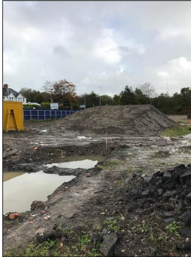
Photograph 8. Exposed earth (Bare ground archaeological dig site)
