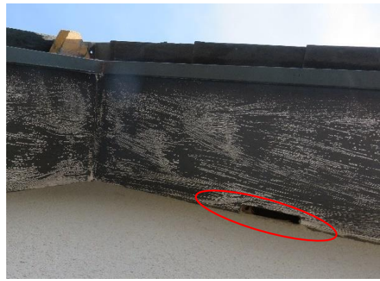
Plate 12: Bat access slot
