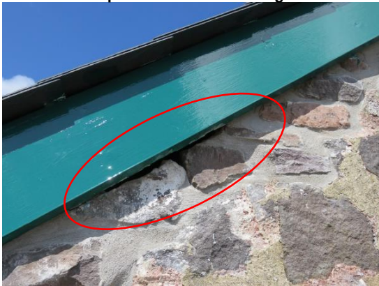
Plate 11: Example of bat access slit at gable wall fascia
