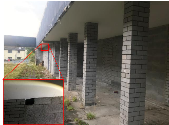
Plate 10: Blocked doorways of south side of Upper Building, possible emergence location
