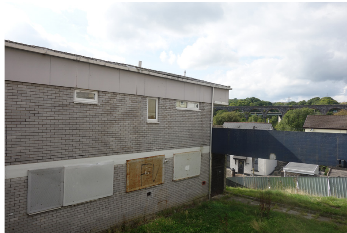
03) View towards the viaduct
