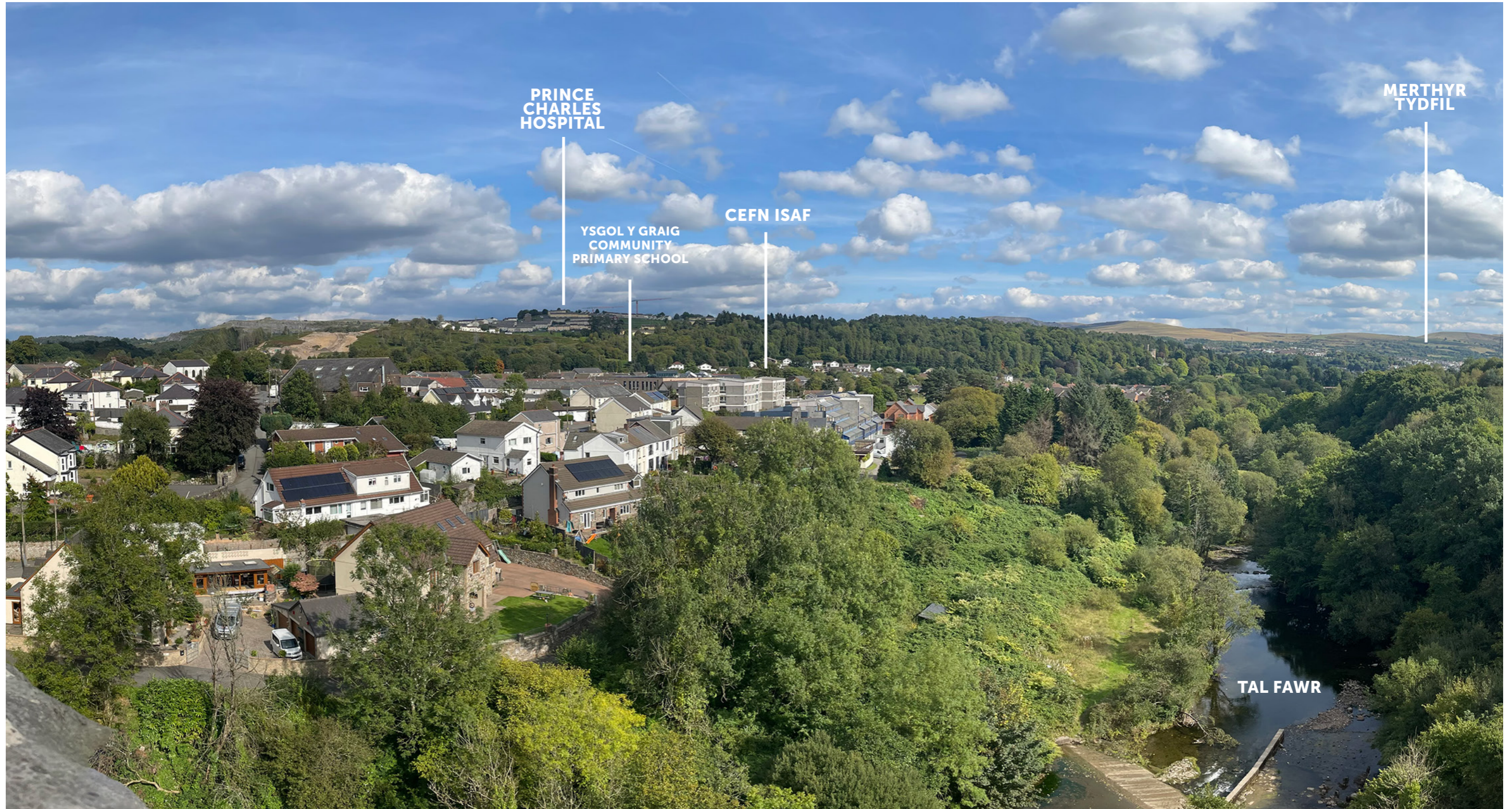
Panoramic view of the site and wider context from the Cefn-Coed viaduct
