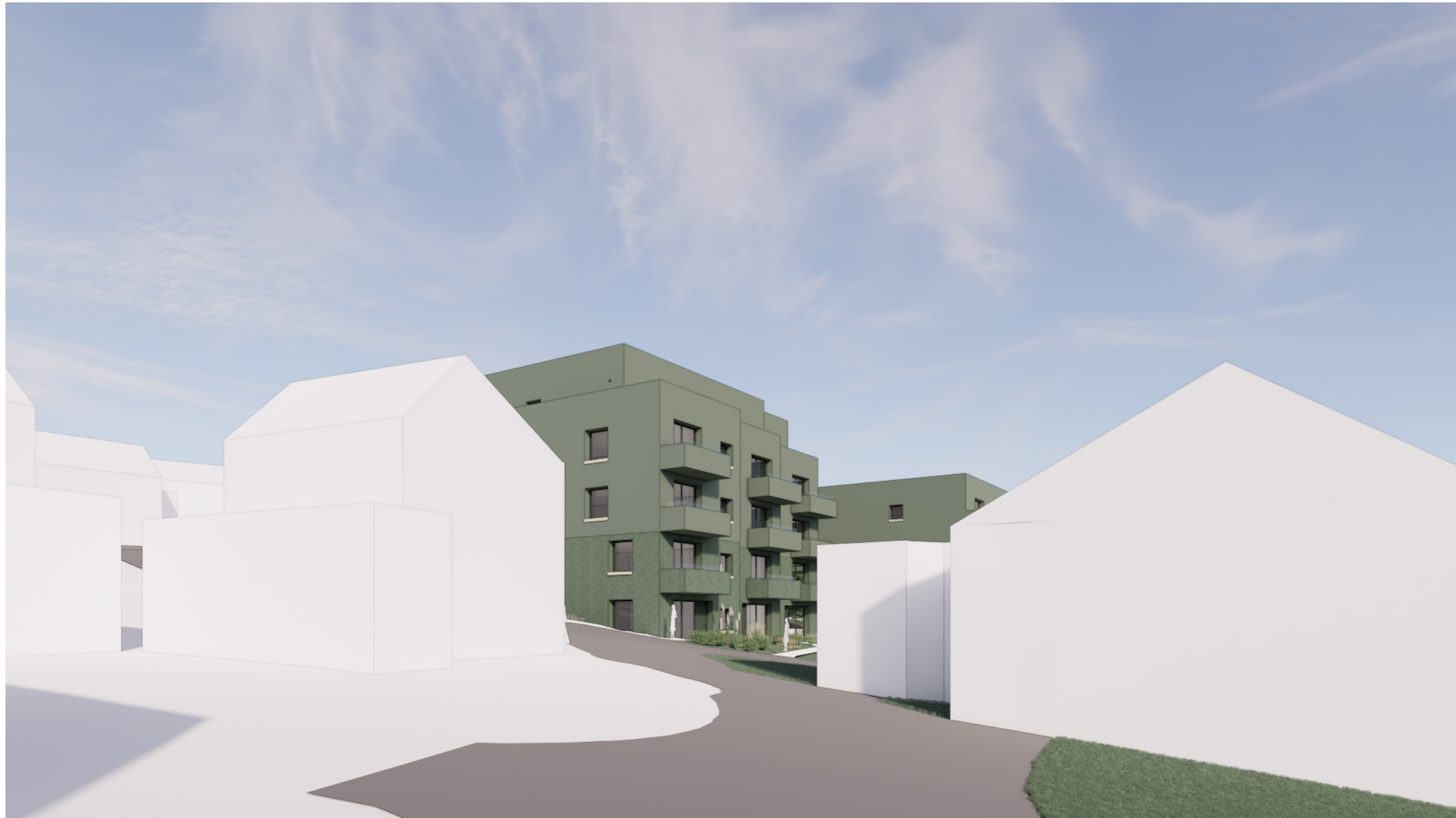
Sketch view looking between houses at the bottom of Wern Road. The top floor of each block is set back to reduce the perceived massing scale.
