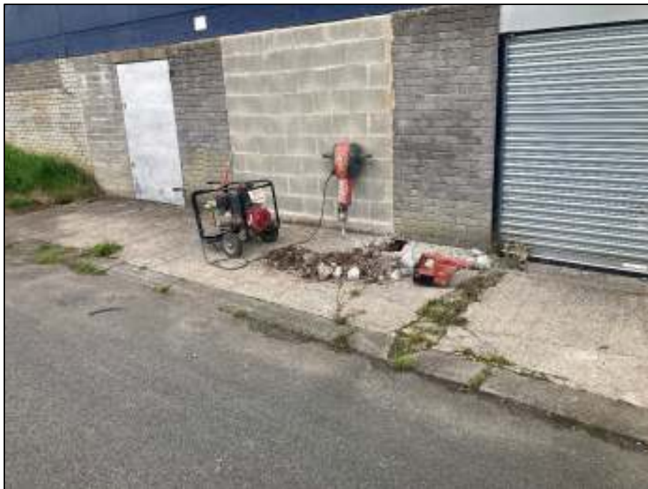
P8: Photograph showing TP05 Location
