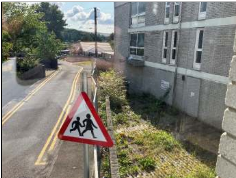
P4: Photograph showing Northern courtyard looking west
