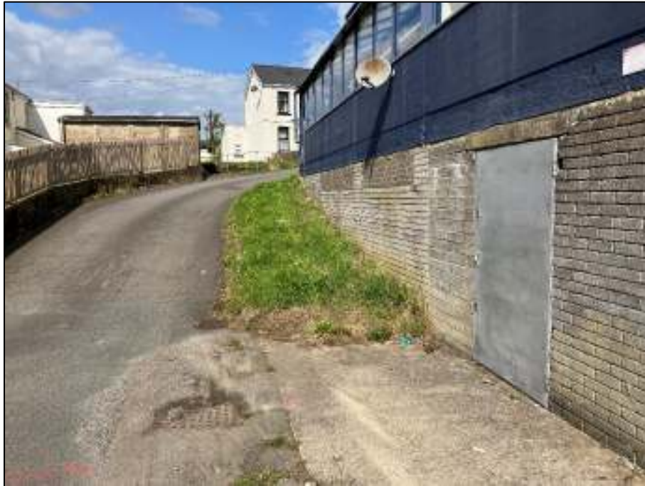
P7: Photograph showing access road running along site western boundary
