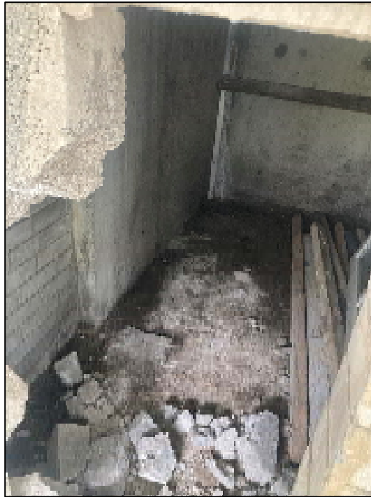
P5: Photograph showing TP03 Location
