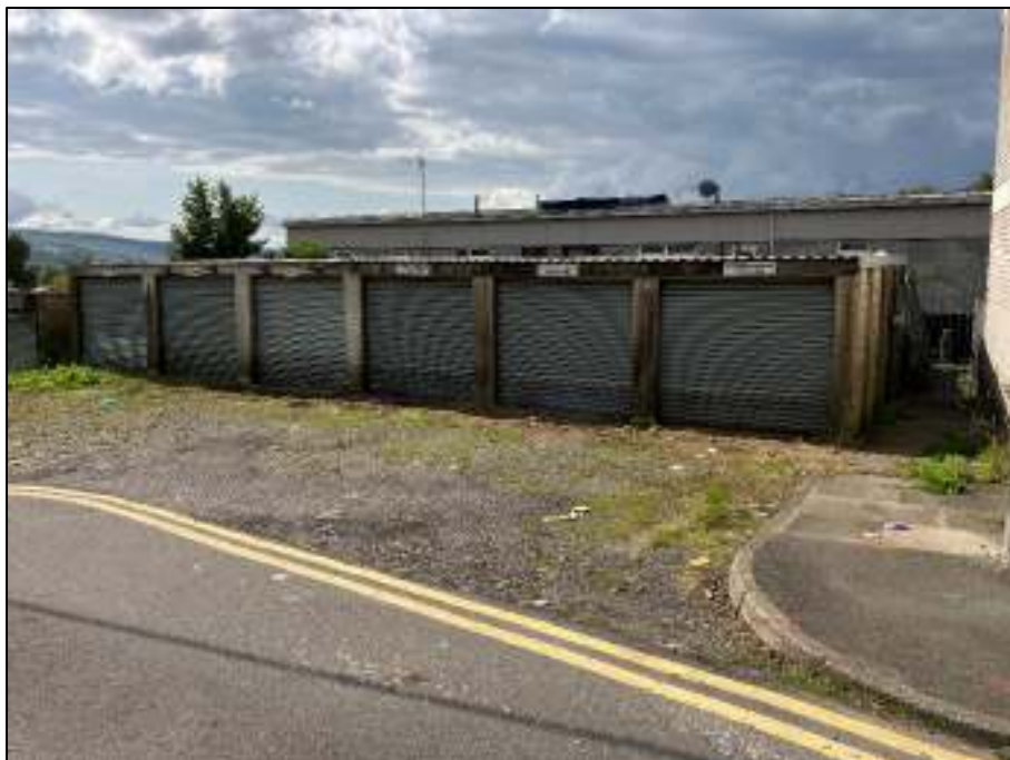
P6: Photograph showing garages located on sites northeastern boarder
