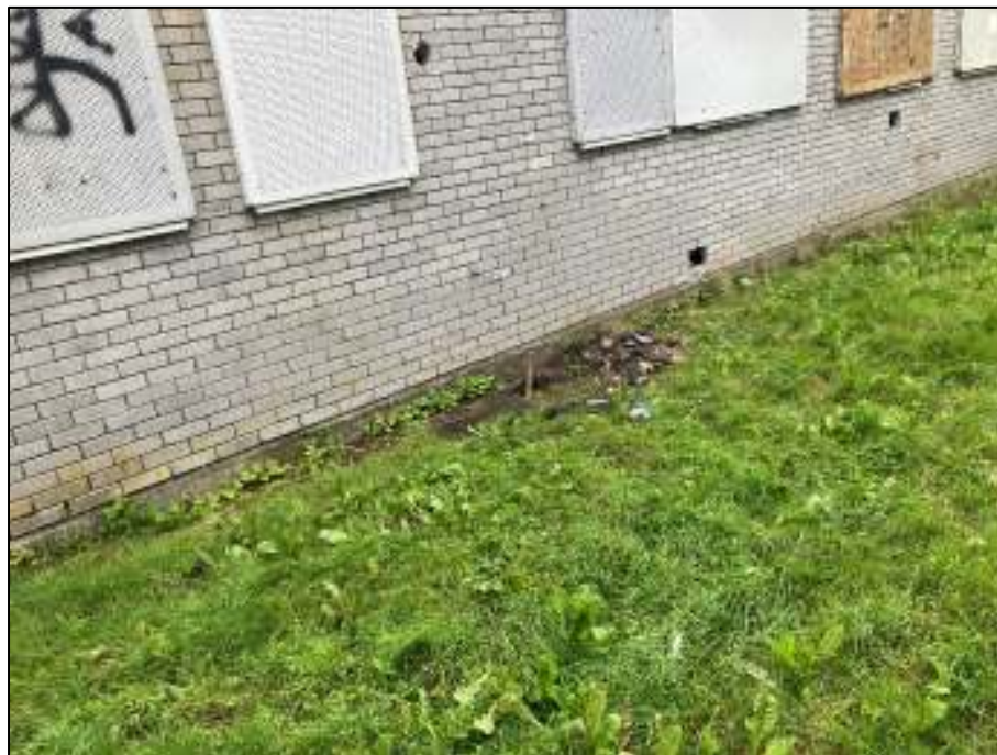
P6: Photograph showing location of TP04
