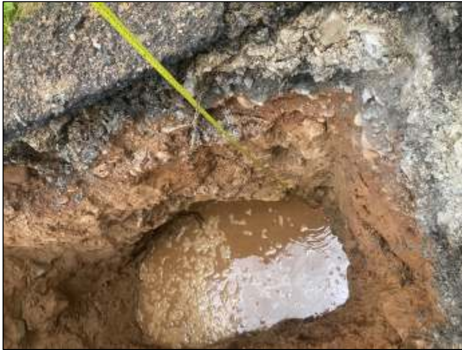
P13: Photograph showing TP08 during soakaway testing
