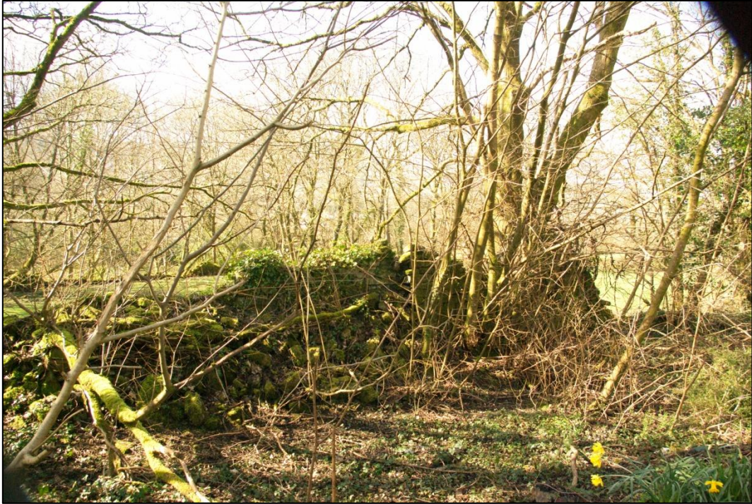
Plate 5: Remains of the ironworks stables in the northern part of the site from east
