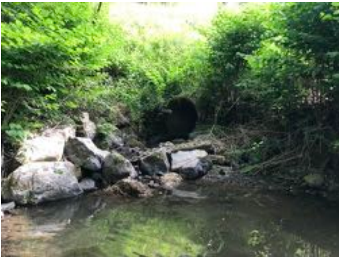
Fig.15 - Culvert where stream enters the site
