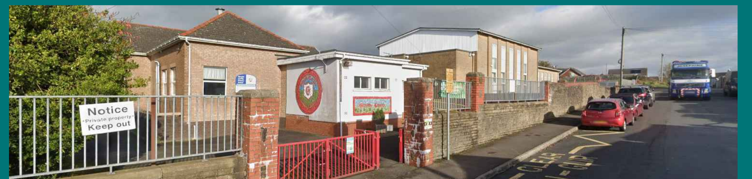
VIEW LOOKING NORTH
